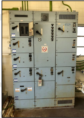
Digester Heat / Mix Room and old MCC
